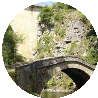
the two bridges
